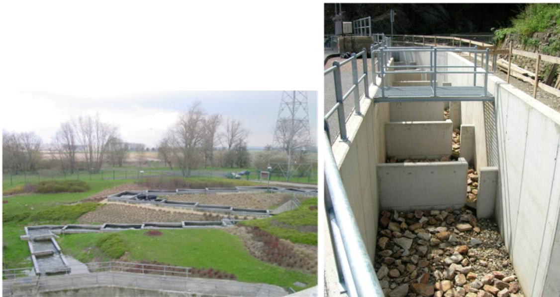
Figure 4: Two examples of fish ladder in Belgium.
